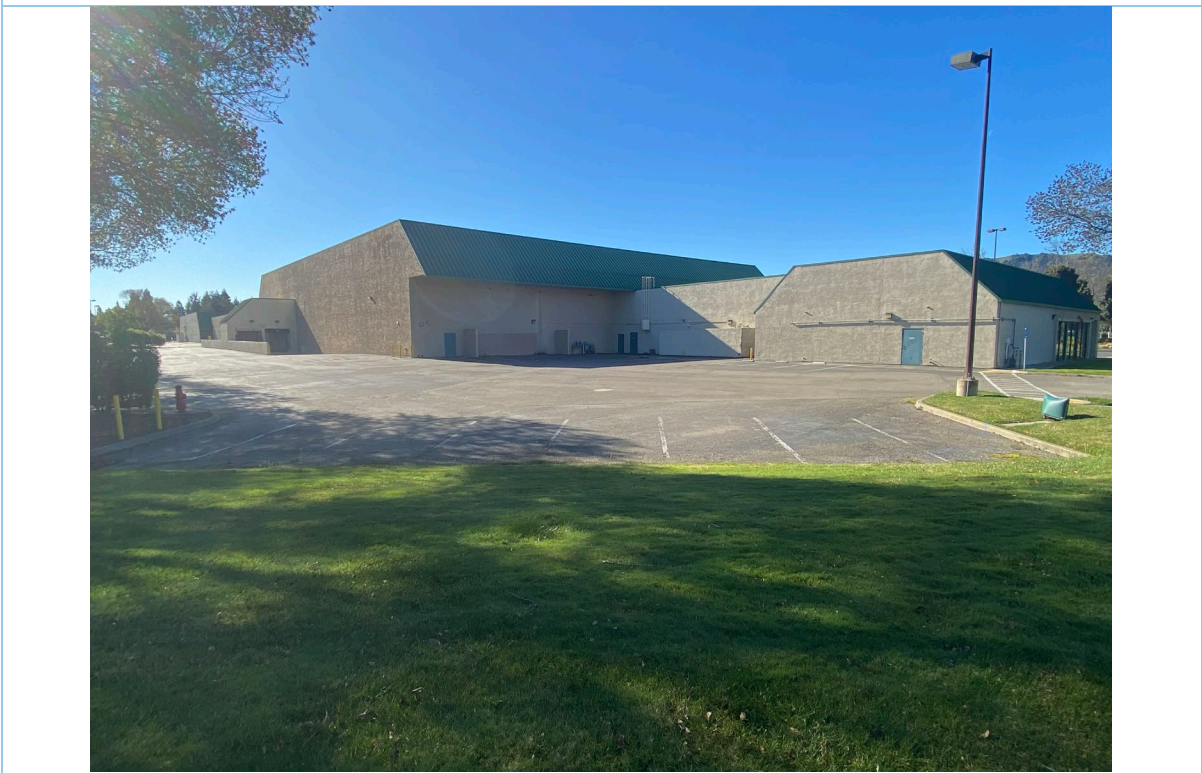
Photograph 2: Overview of the project area from the northeast corner; facing southwest.
