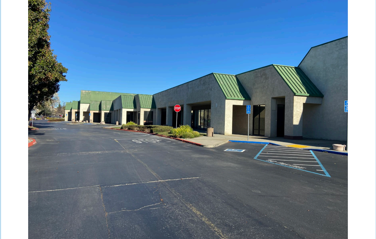
Photograph 5: Detail of eastern building block; facing northeast.
