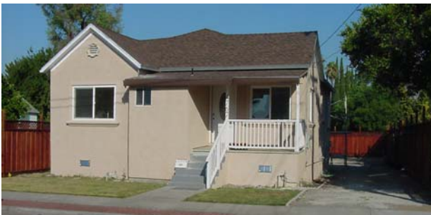
Photograph of existing main structure
