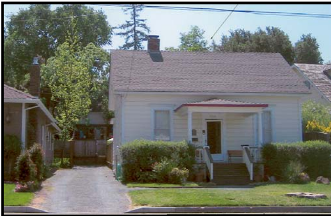
Front of Boyce Residence - Existing
