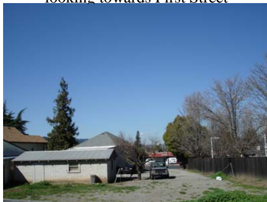
Partial rear view of the subject site looking towards First Street
