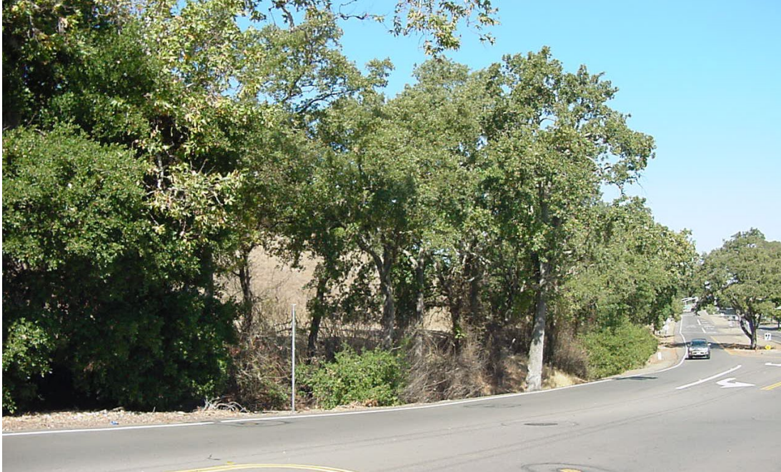
Figure 11: Section of Foothill Road where creek must be filled for bike lane.
