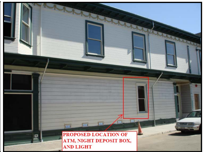
Figure 4-Division Street Elevation (photo taken 9/5/08)
