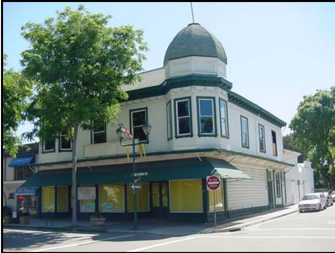
Figure 1-Buildings Prior to the Renovation and Addition
