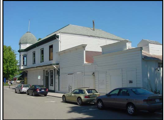
Figure 2-Buildings Prior to the Renovation and Addition
