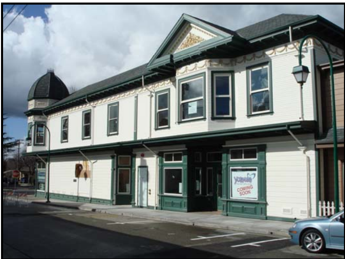
Division Street Elevation of Buildings 1 and 4
