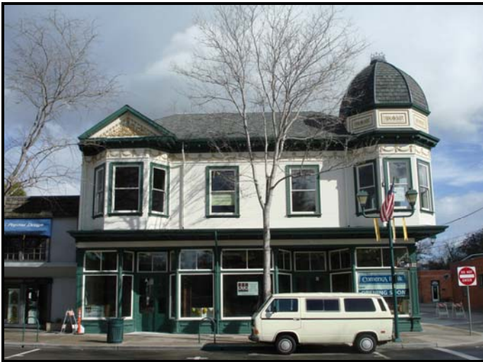
Main Street Elevation of Building 1
