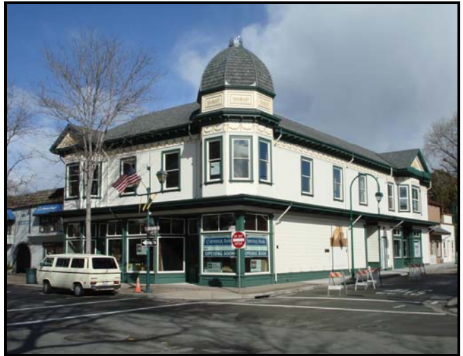
Main Street/Division Street Corner Elevation
