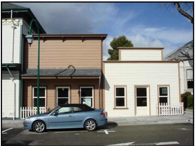
Division Street Elevation of Buildings 2 and 3
