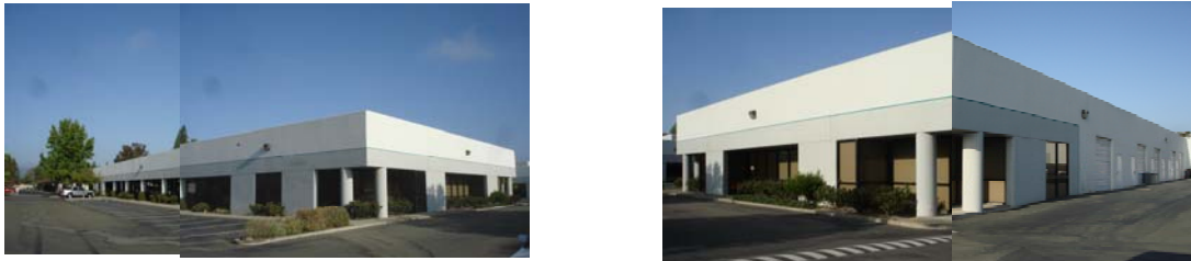
Figure 1.2 – 3: Photos of the exterior of 1249 Quarry Lane, Suite 150
