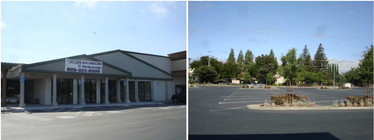
FIGURE 2: PHOTOS SHOWING THE SUBJECT TENANT SPACE AND A PARTIAL VIEW OF THE PARKING LOT
