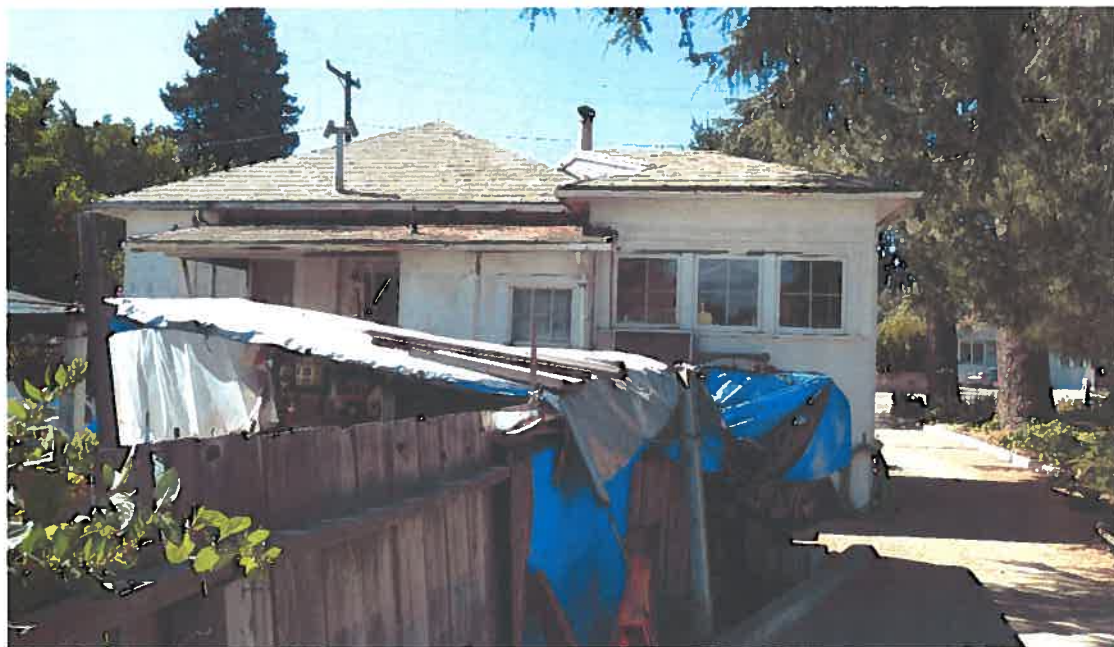
View of rear (north) façade, July 16, 2010 (Architectural Resources Group)
