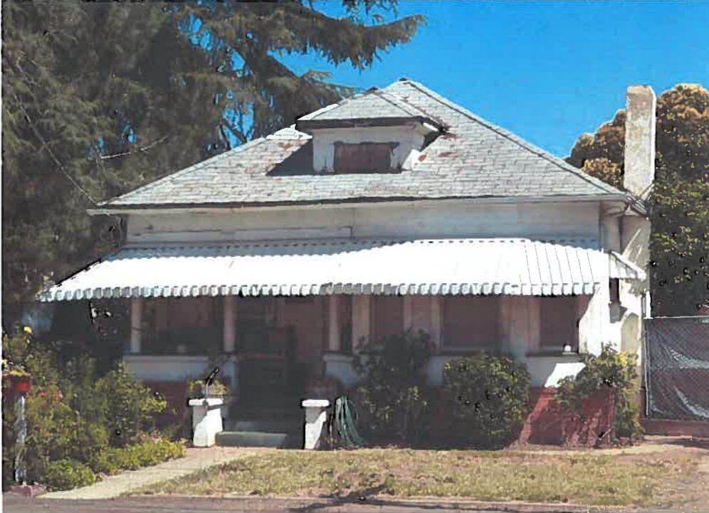
View of primary (south) façade, July 16, 2010 (Architectural Resources Group)
