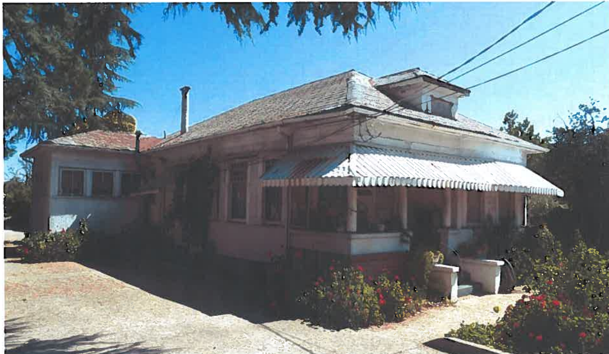
View of west and south façades, July 16, 2010 (Architectural Resources Group)
