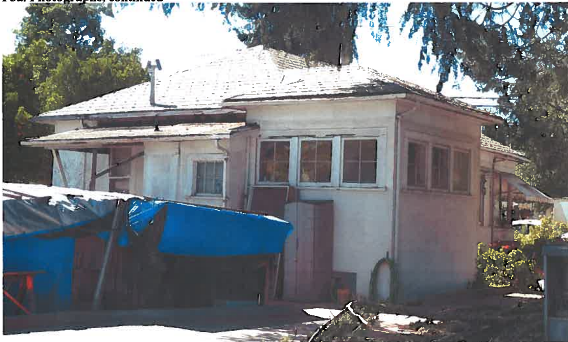
View of rear (north) façade, July 16, 2010 (Architectural Resources Group)
