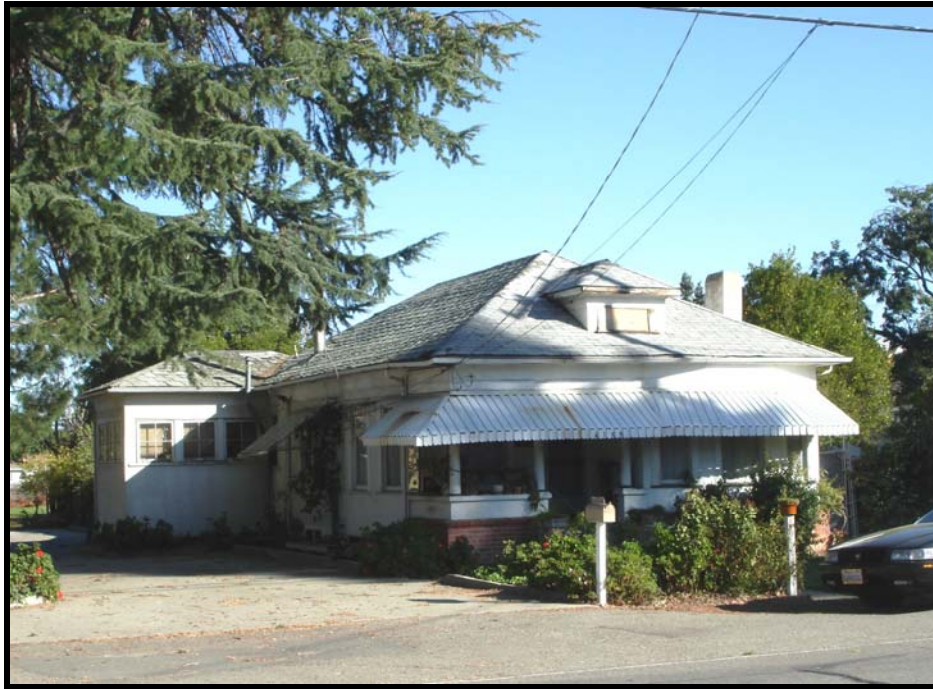
2010 Photograph of the Existing House at 4189 Stanley Boulevard
