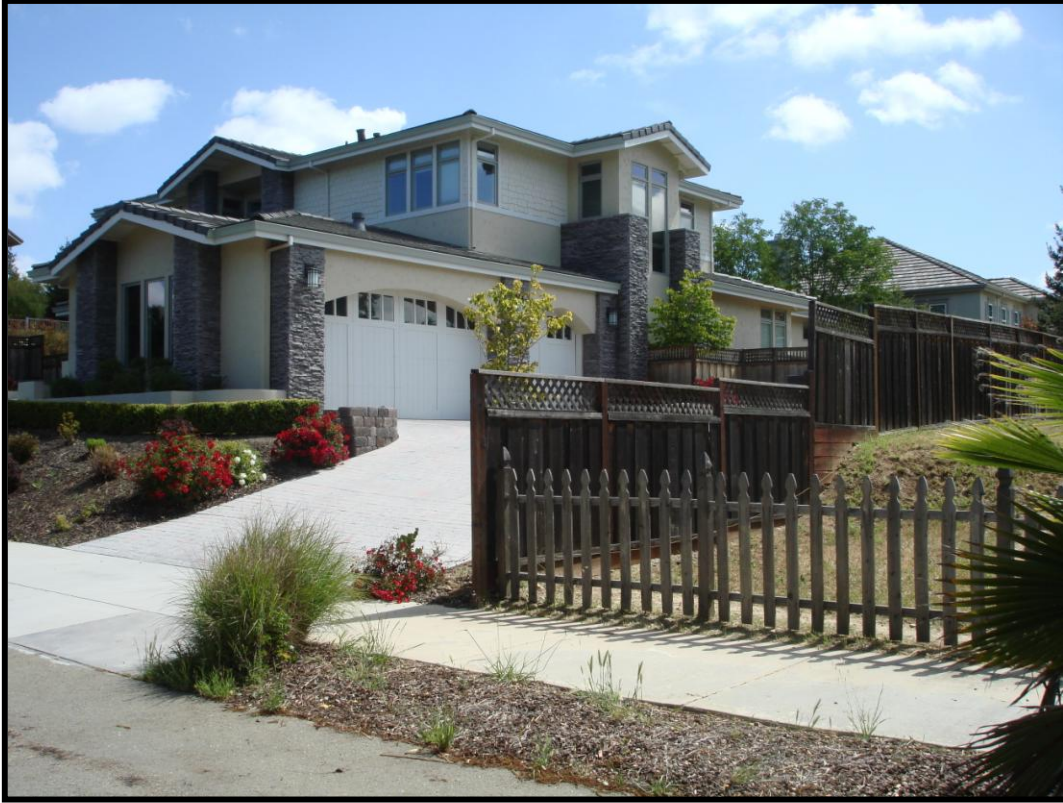
Figure 7: Existing home on the east side of Sycamore Terrace.
