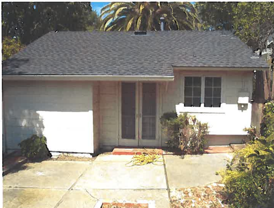
Rear elevation of 205 Neal St., viewed facing northeast.
