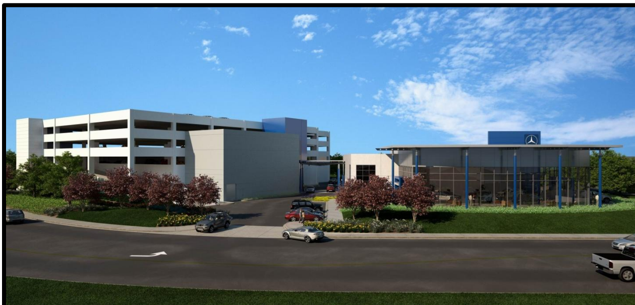
FIGURE 8: Rendering showing showroom facility and service facility/parking structure as viewed from Owens Court
