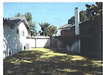
Partial view of existing east side elevation and rear/side yard
