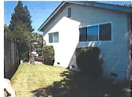
Partial View of Subject Property's Rear Elevation and Rear Yard
