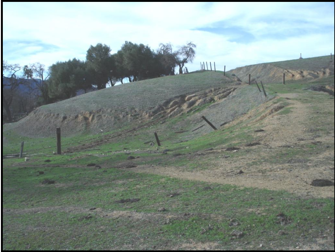
Figure 10: Road Cut and Dam.
