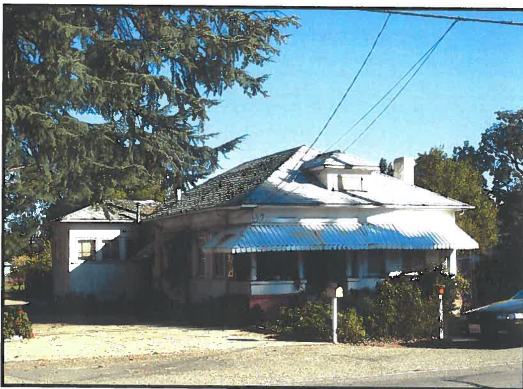
Figure 1: 2010 Photograph of the Existing House at 4189 Stanley Boulevard
