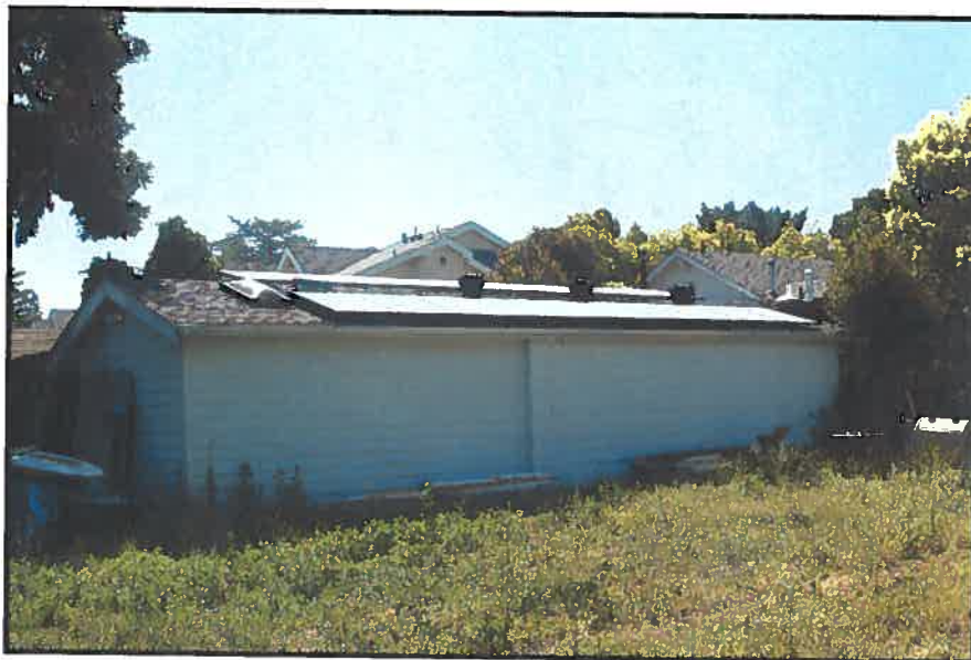
Figure 6: PV Panels at 4151 Stanley Boulevard
