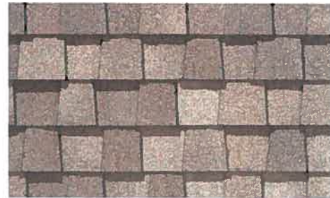
9 Composition Shingle Roof
