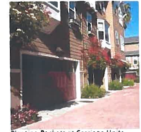
Planting Pockets at Carriage Units
