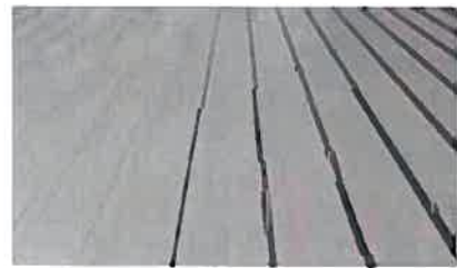
1 Standing Seam Metal Roof
