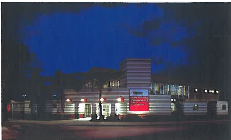
Cloverfield Services Center – Emergency Shelter by OPCC in Santa Monica, CA Photo courtesy of OPCC in Santa Monica
