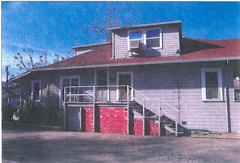
East façade showing entrance door to second floor unit and stairs. View to west
