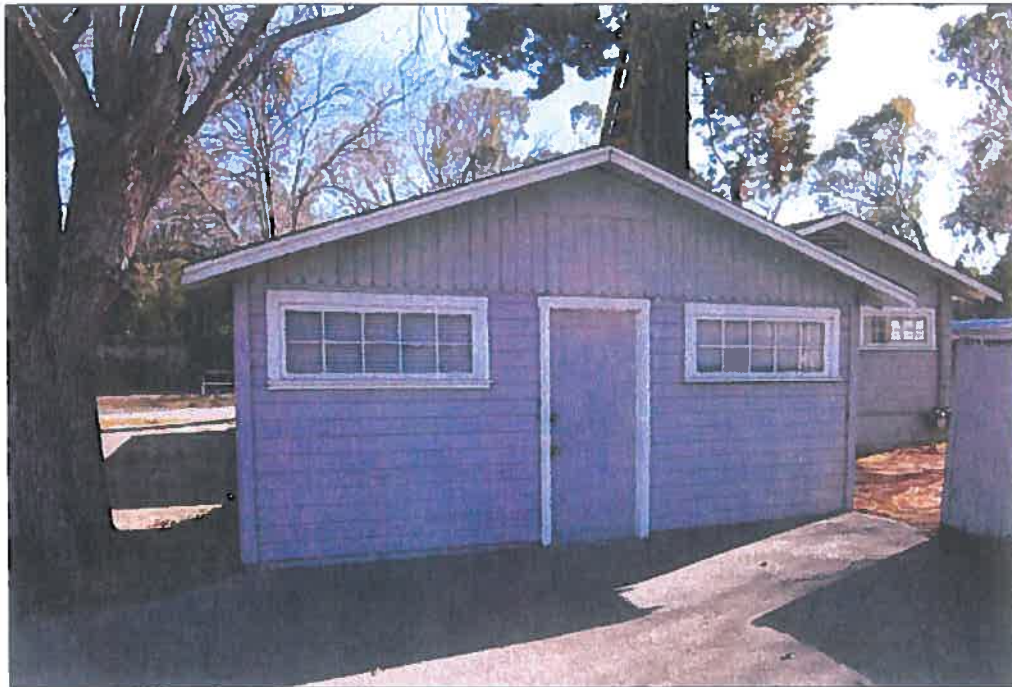
View of front façade of storage building. Laundry room at rear of small residence is visible at right. View to east
