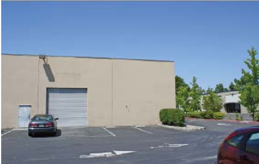
Existing Site Exterior
