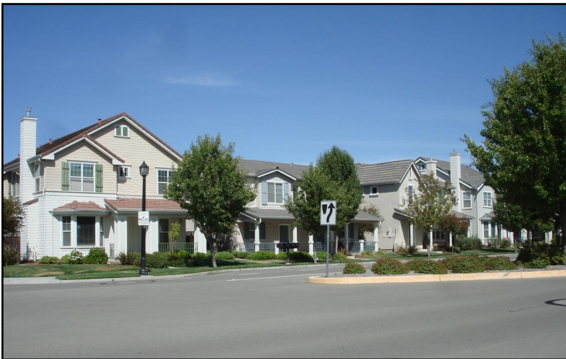
Figure 5: Walnut Hills Development from the West Side of Valley Avenue.
