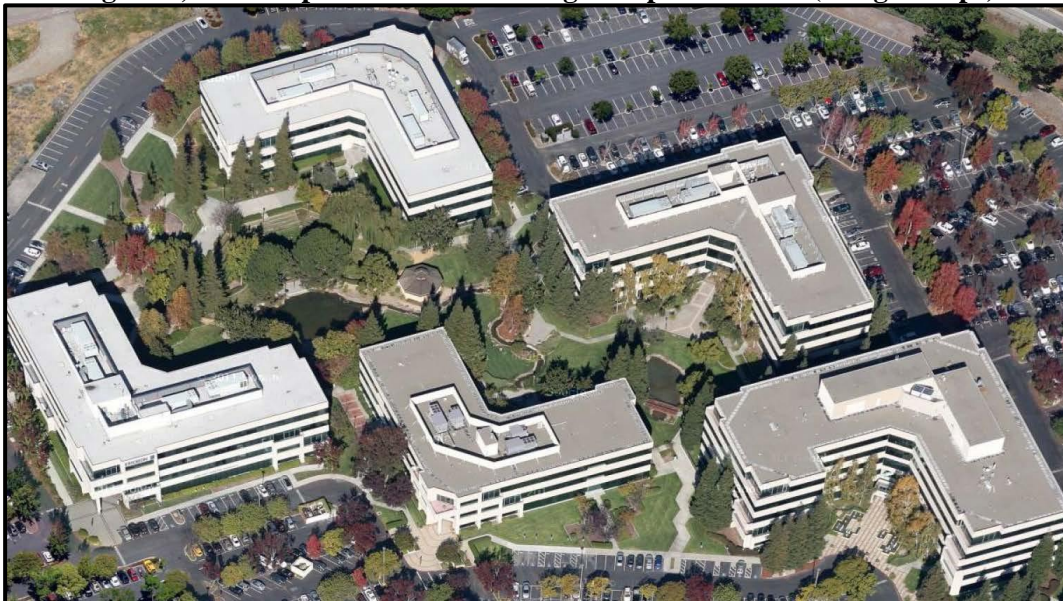
Figure 9, Landscaped Area at Stoneridge Corporate Plaza (Google Maps)
