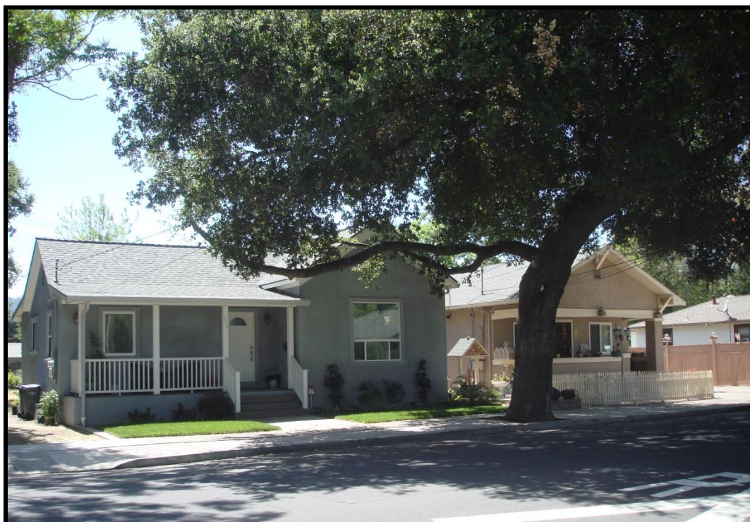
Figure 1, Photograph of Existing Home from Rose Avenue
