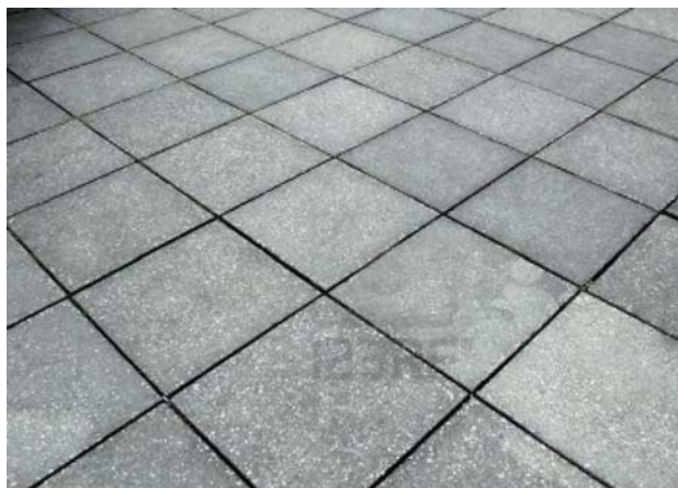
Enhanced Concrete Paving
