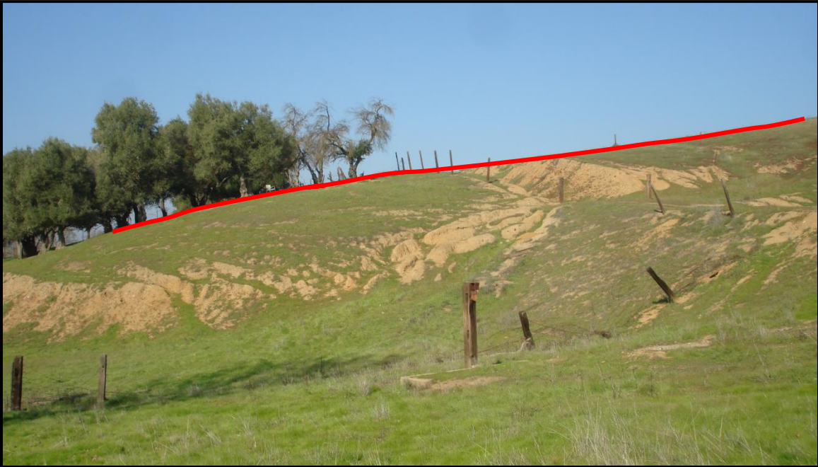
Figure 9: Existing Cut and Slope
