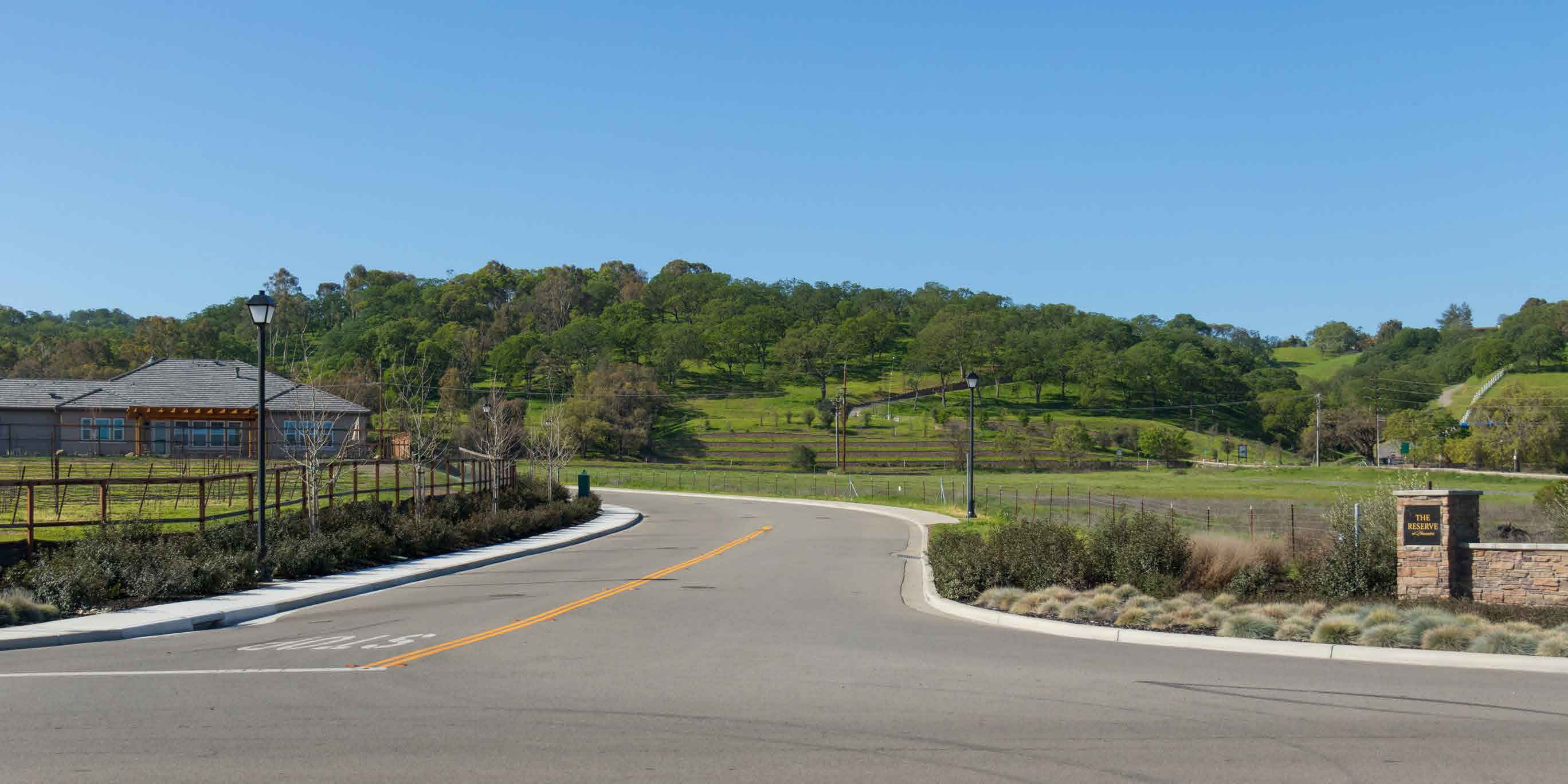
VIEW B - EXISTING SITE PHOTO VINEYARD AVE AT MANOIR
