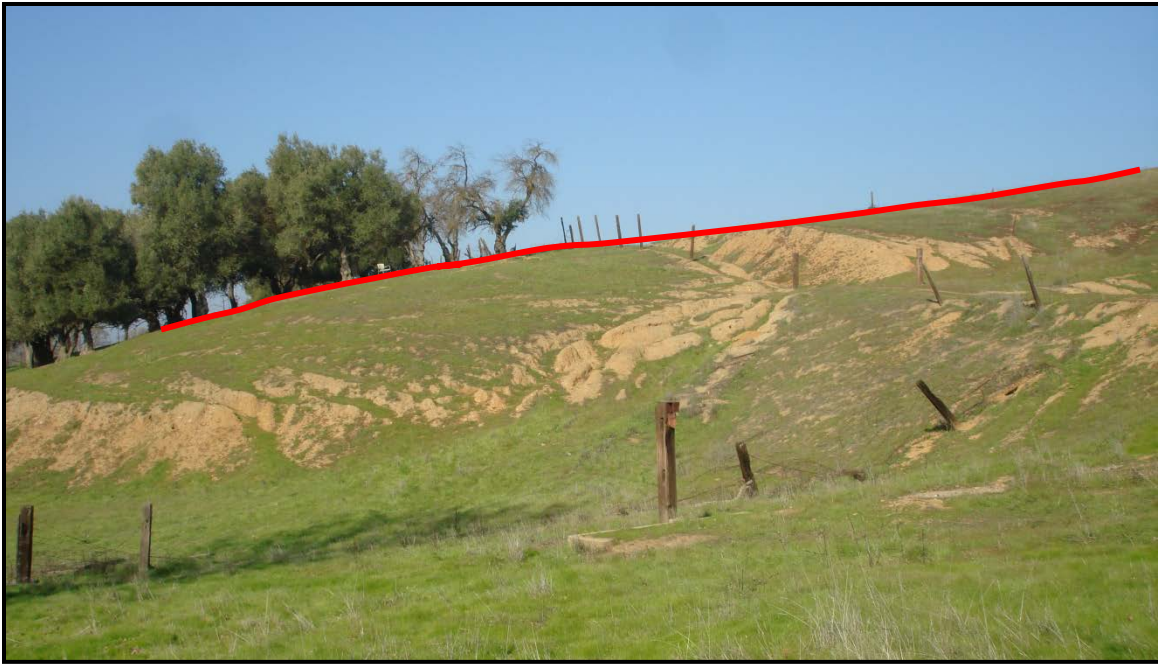
Figure 8: Existing Cut and Slope
