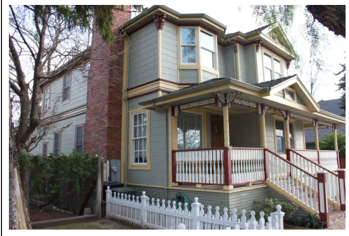
Looking SE from First St.
