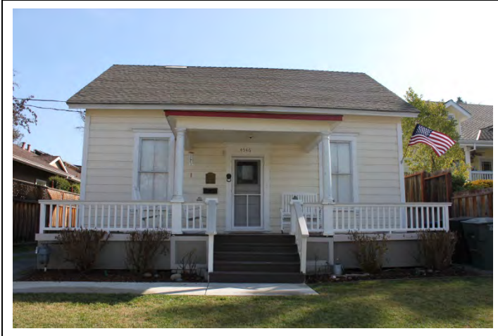
Looking E from Second St.
