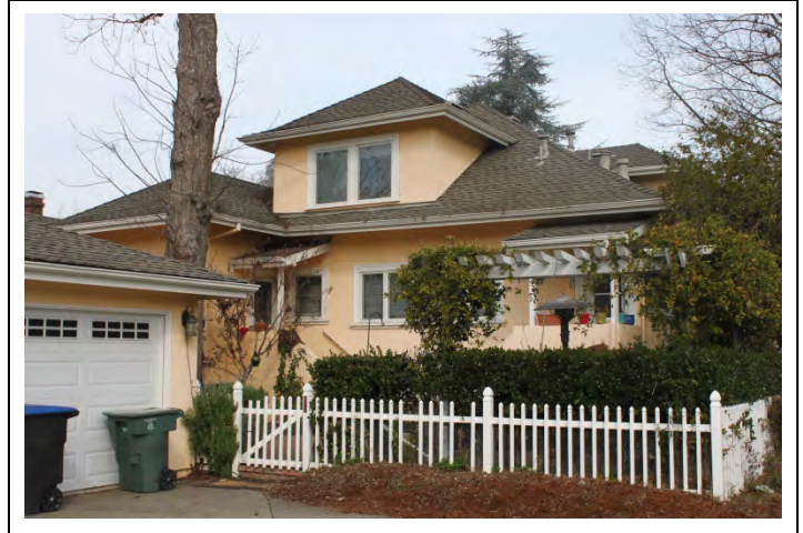
Rear elevation, looking NW from Second St.
