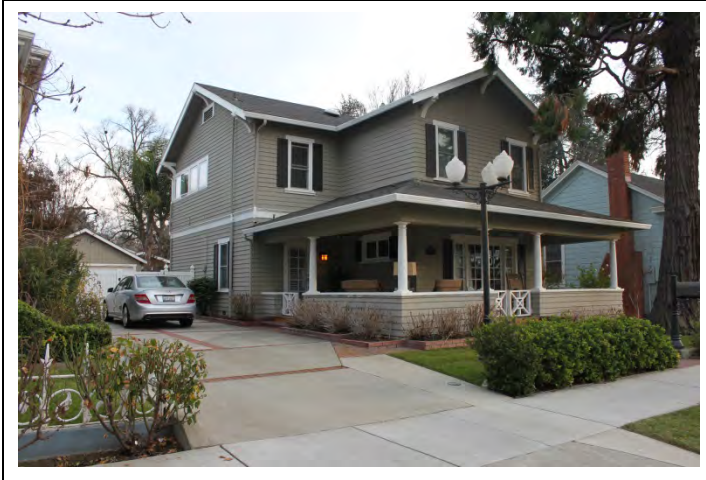
Looking SE from First Street Possible sleeping porch windows visible on second story
