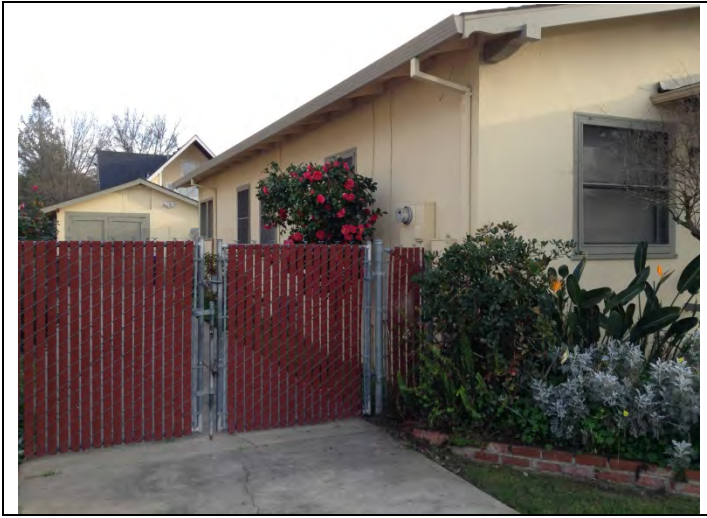
North elevation, looking SE from First Street
