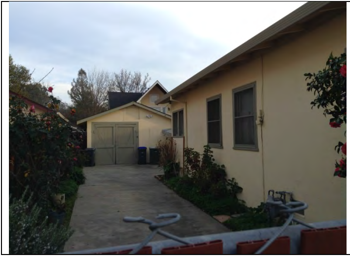
Garage at rear of lot
