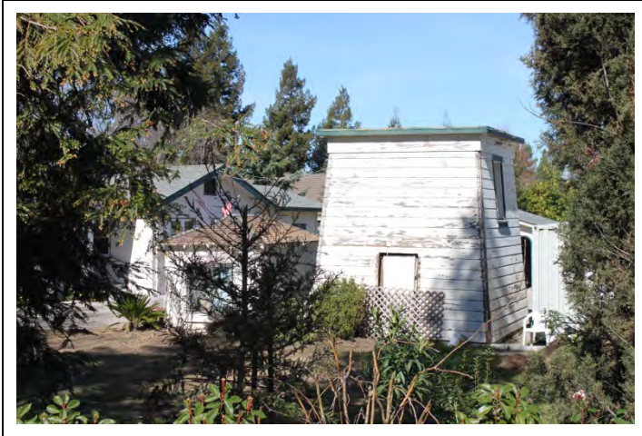
Looking NW from Stanley Blvd. Tank house base and chicken coop
