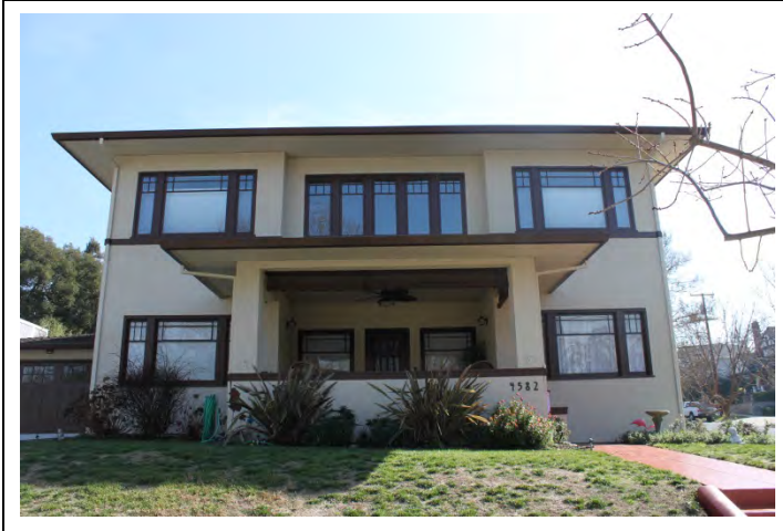
Looking E from Second St.
