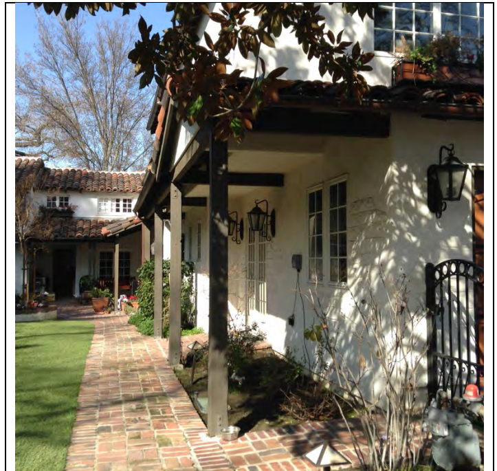
Looking W along 1997 addition
