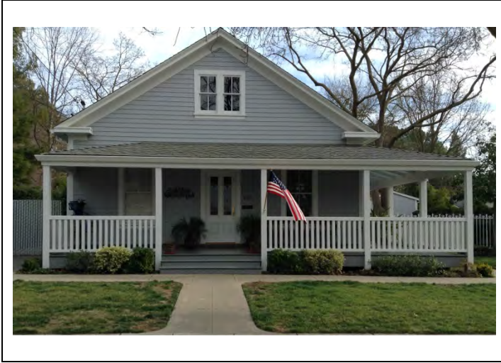
Looking E from Second St.
