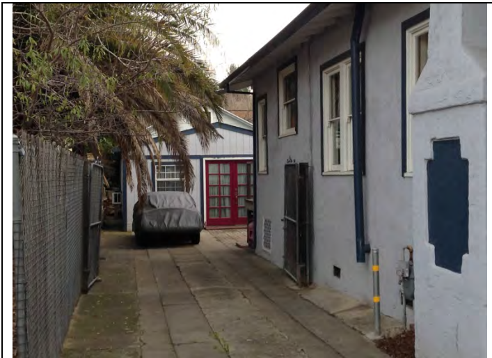
Garage at rear of lot
