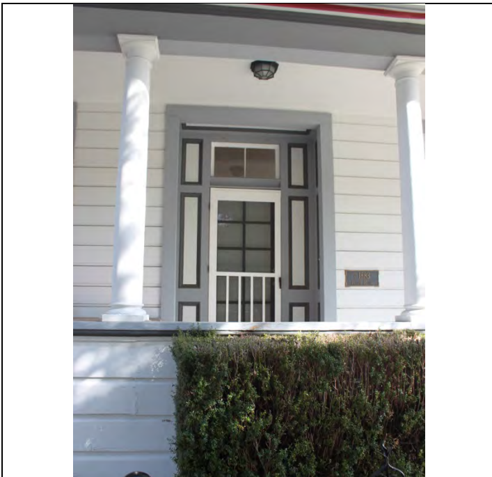
Original main entrance on south elevation
