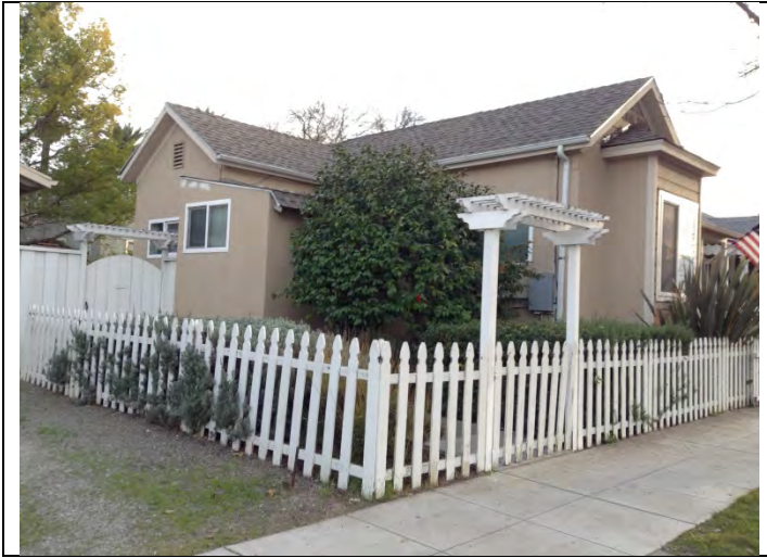
Looking SE from First Street showing enclosed porch
