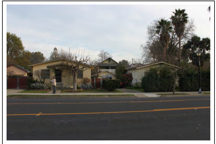
4358 (left) and 4366 (right) First Street Looking E from First St.
