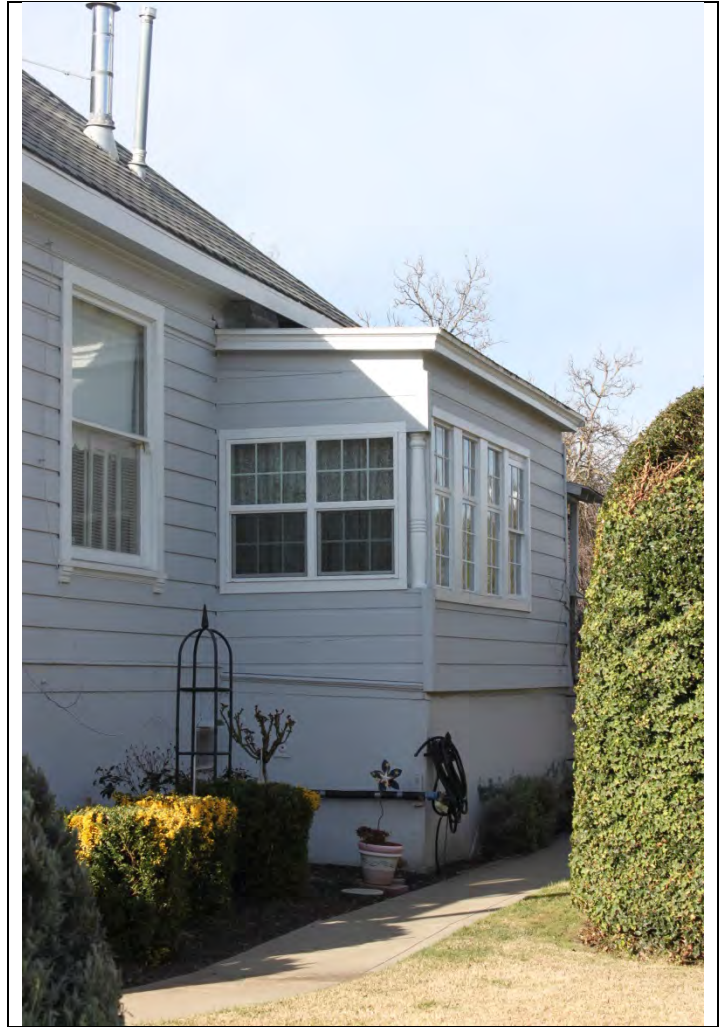
Detail, east porch enclosure with post
