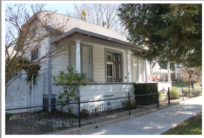
Original main elevation fronting on E. Angela St. Looking NE from E. Angela St.
