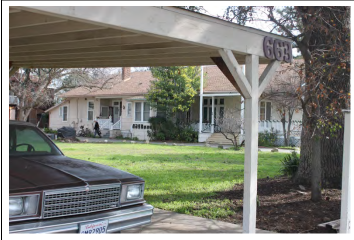
West elevation, looking NE from Rose Ave.
