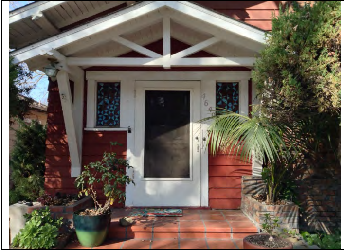
Detail, main entry
