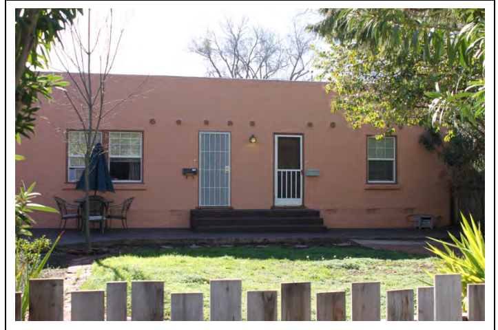
Detail, courtyard, looking S
