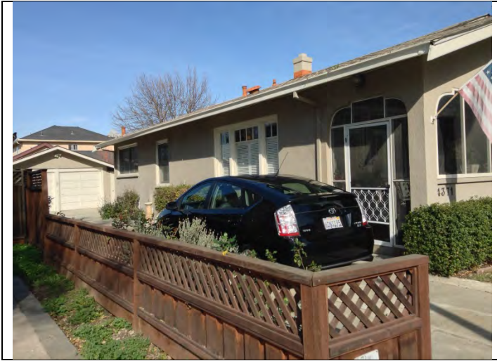
Looking NW from Second St.
