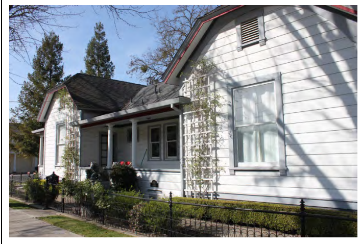
East elevation on Second St. Looking SW from Second St.
