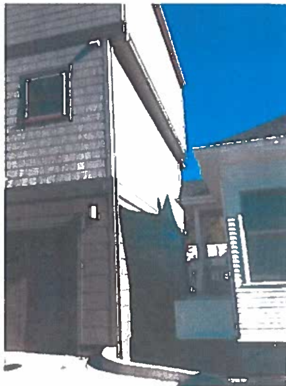
3 story to 1 story architectural scale conflict
