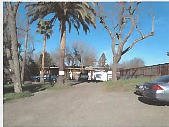
VIEW OF (E) STRUCTURE
