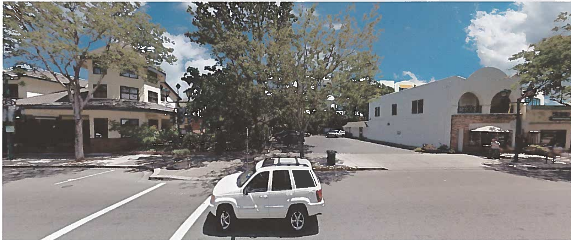
VIEW LOOKING E
