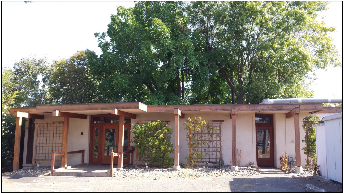
Figure 9: Existing Building to be Demolished
