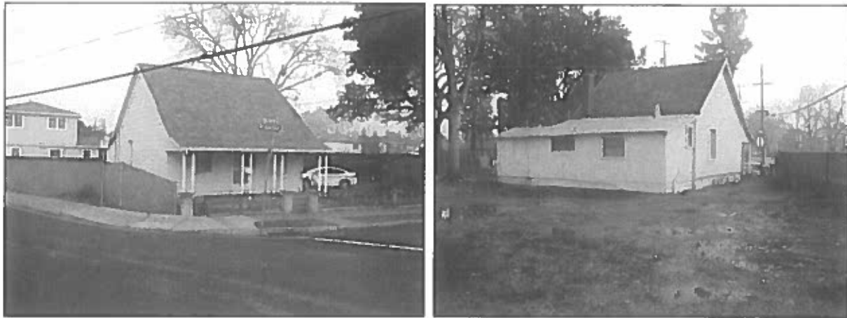
Figures 2 and 3. Left image shows the front and left side elevations of the residence. Right image shows the residence's rear elevation, with a poorly built and full-width rear addition.
