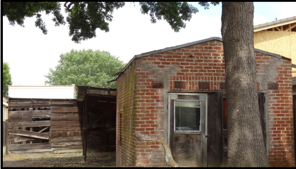
Figure 3: Accessory Structure and Carport
