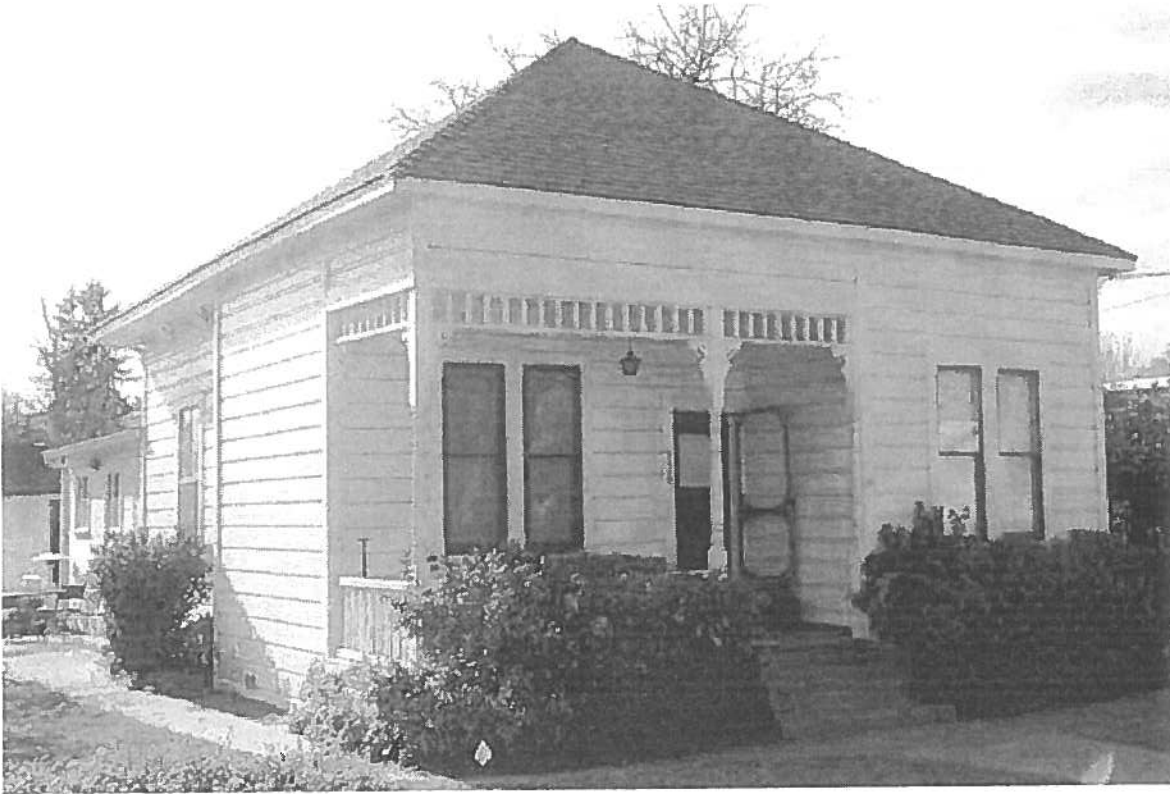
Fig.2 – 536 St. John St. - Left (east) side and Front (with non-historic porch addition at far left)
