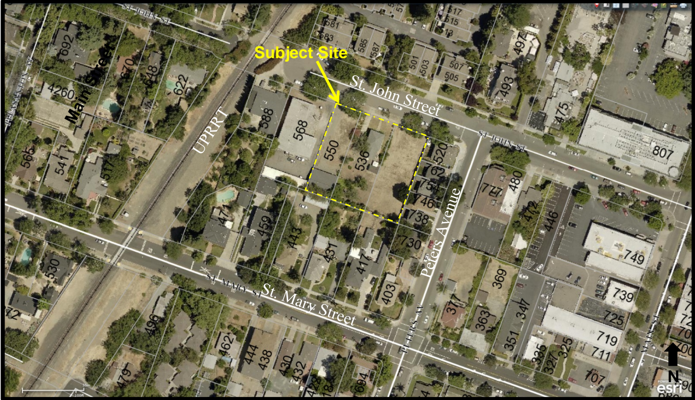
Image 1: Aerial View of the Project Site
