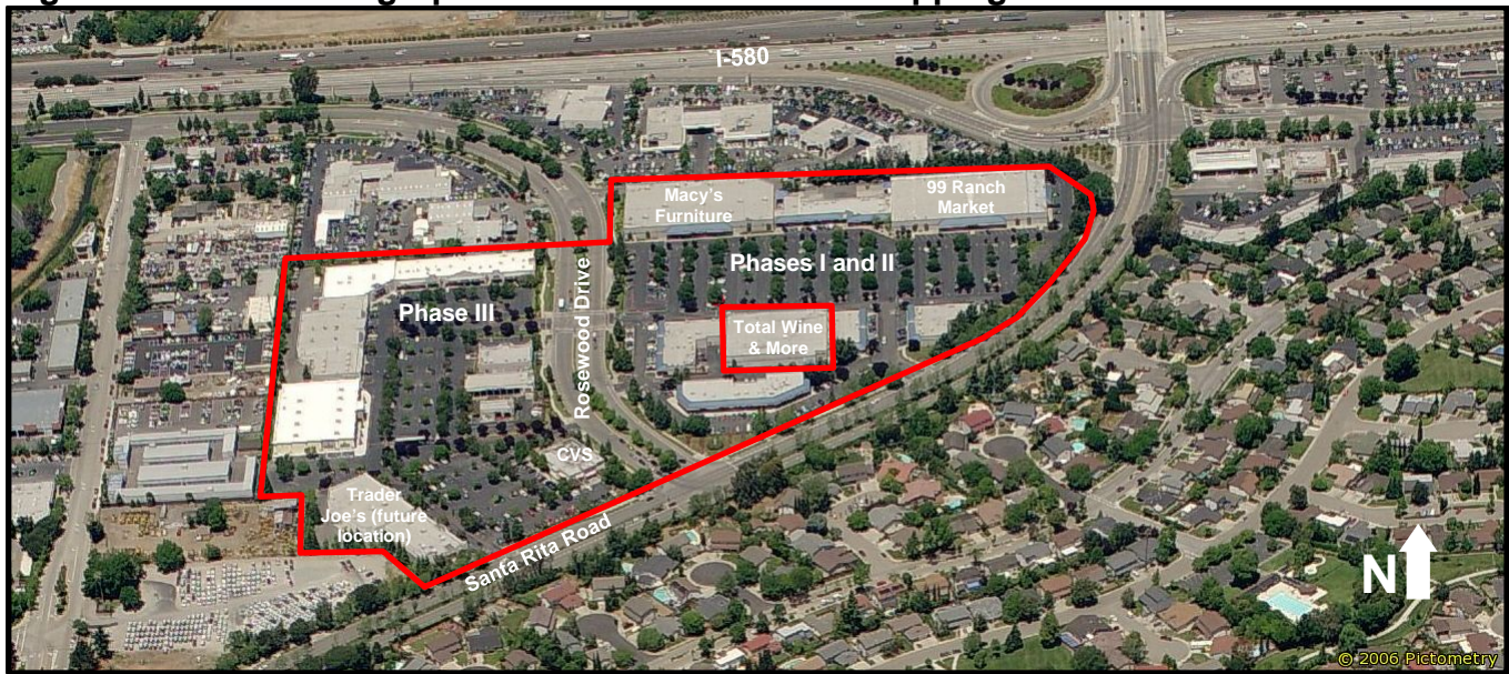
Figure 1: Aerial Photograph of The Rose Pavilion Shopping Center
