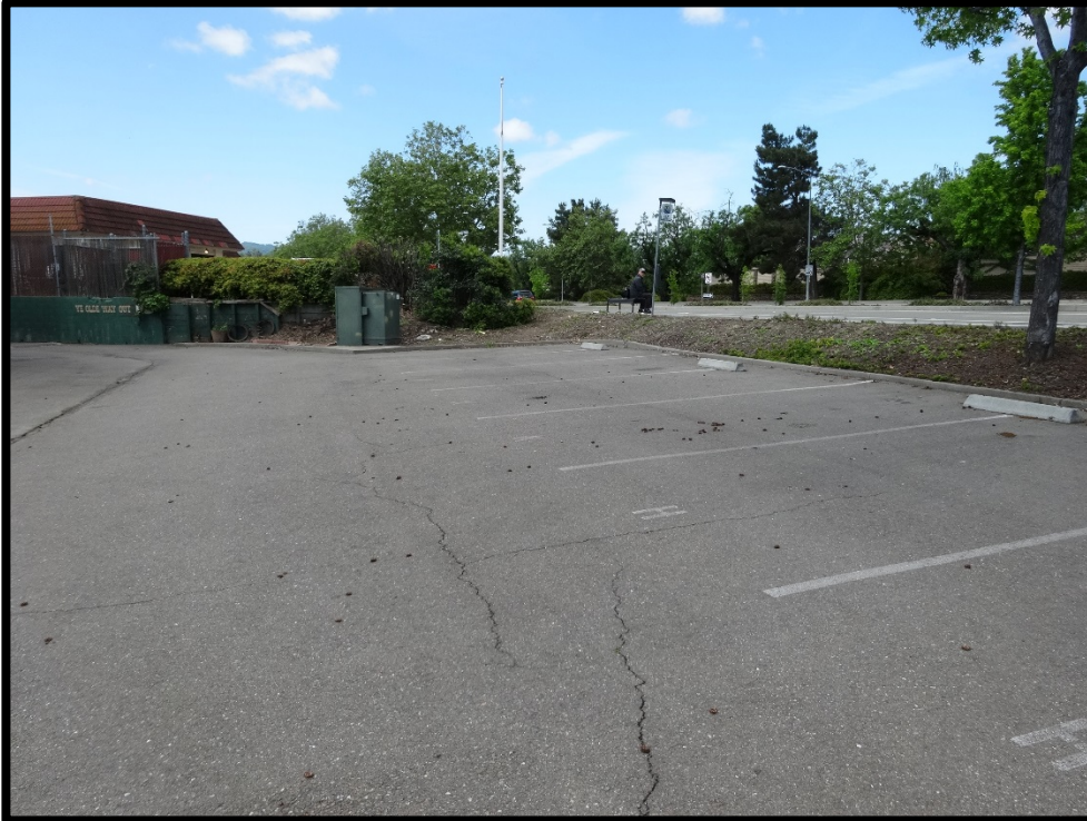
Figure 4: Parking Area Adjacent to Stanley Boulevard
