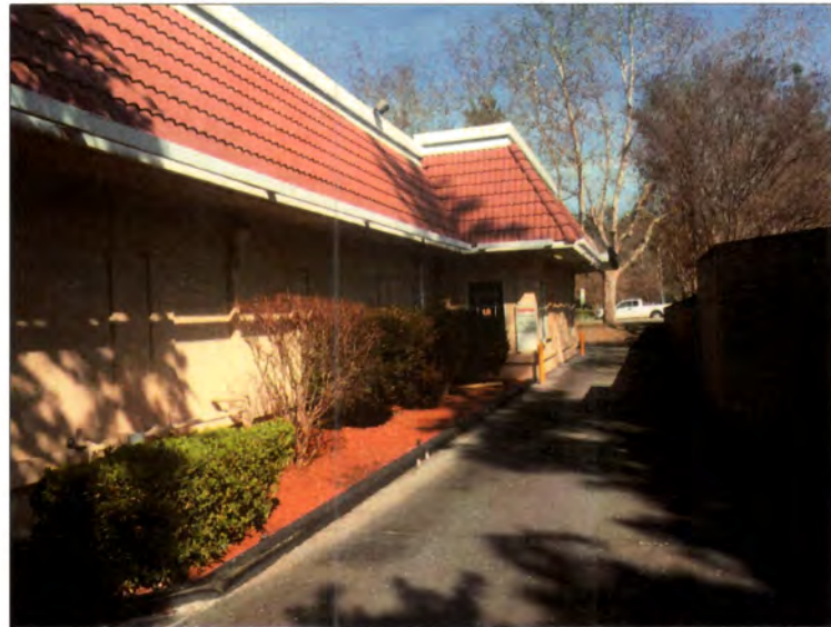
BLDG. PHOTO @ LEFT SIDE 7
