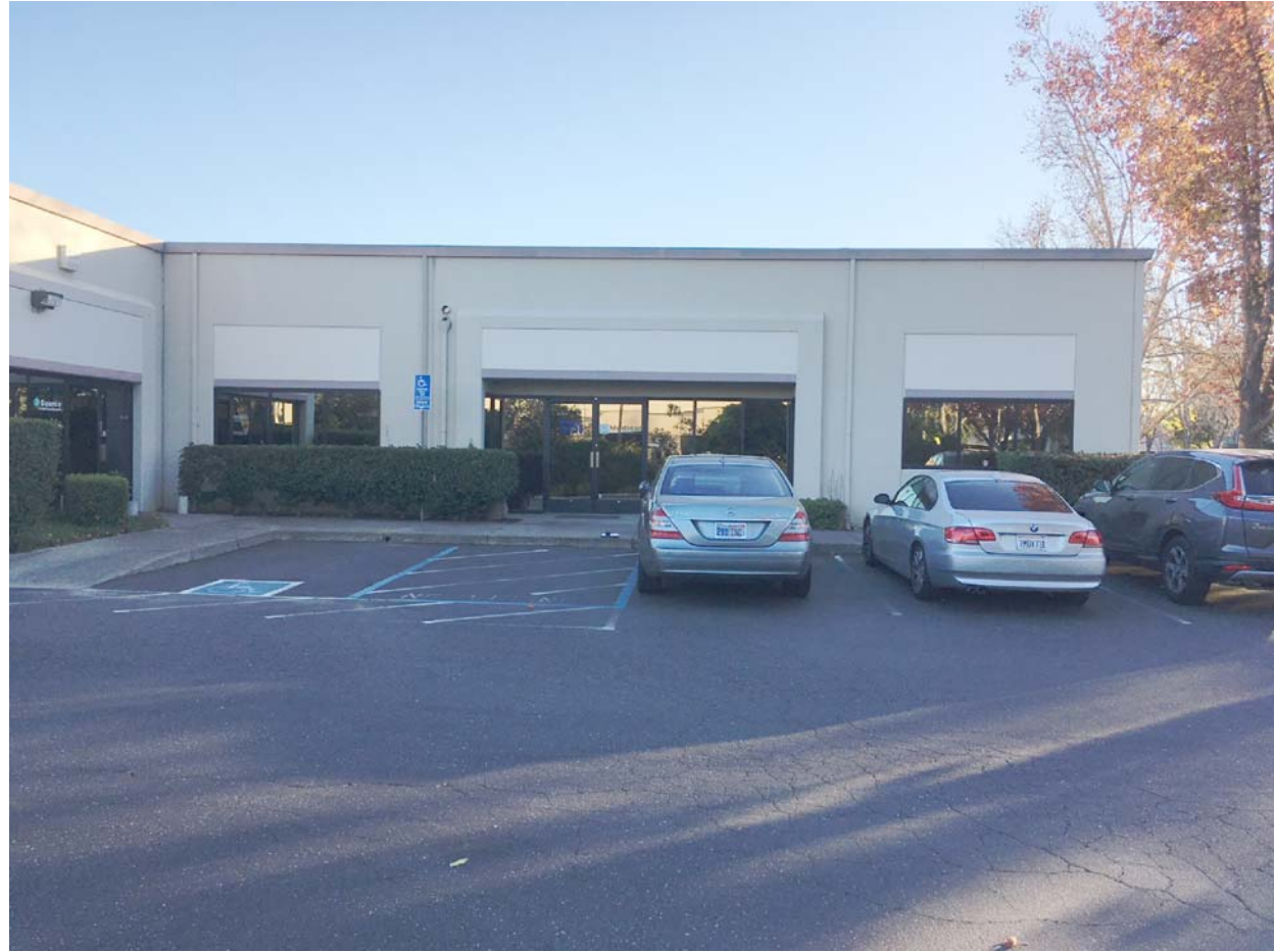
EXISTING BUILDING NORTH ELEVATION VIEW (MAIN ENTRANCE)
