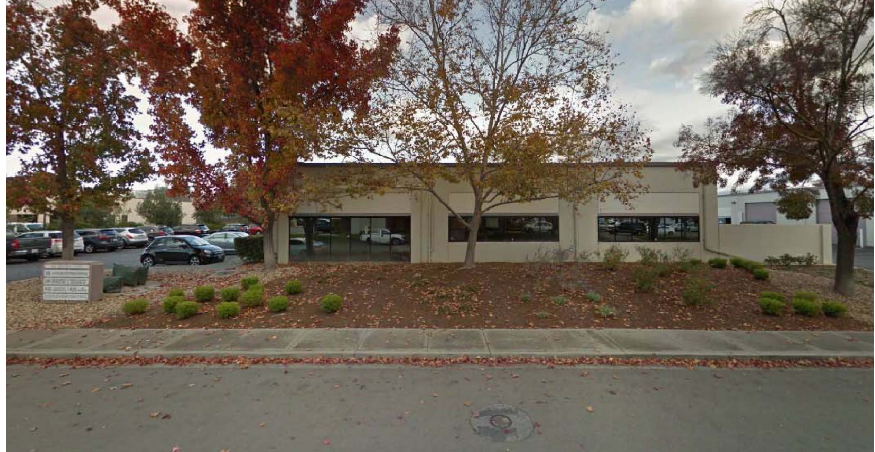
EXISTING BUILDING WEST ELEVATION VIEW (QUARRY LANE VIEW)
