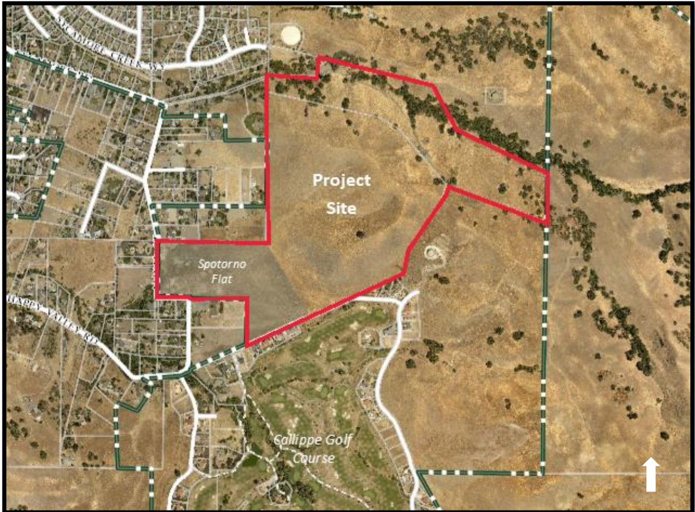
Figure 1: Aerial of Project Site and Surrounding Uses
