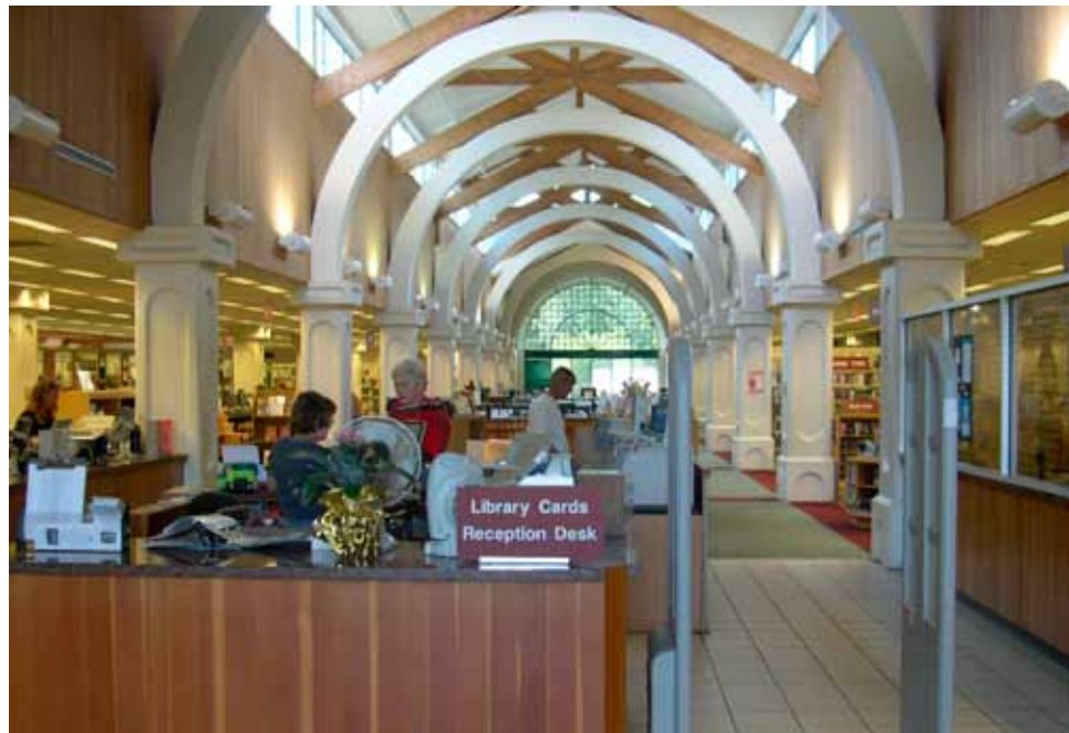
FIGURE 2-2 Existing Pleasanton Library, main entrance
