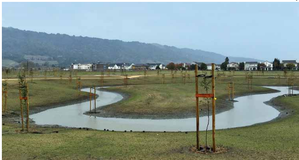
FIGURE 2-11 Bio-swale for stormwater management
