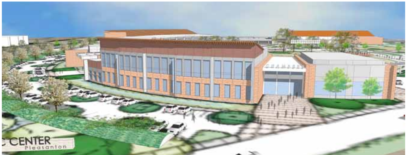
FIGURE 7-12 Detail entry view at City Hall and Council Chambers
