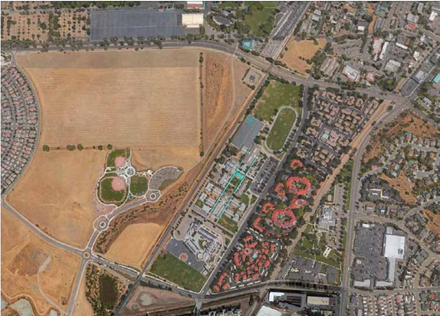
Aerial view of Bernal Park and the downtown site
