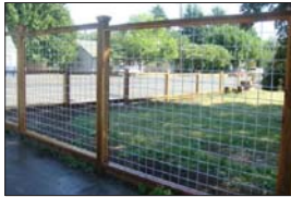
6' WELDED WIRE MESH FENCE
