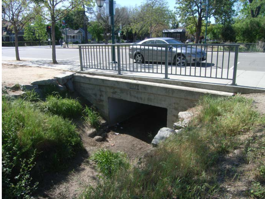
Photograph 2. Culvert No. 2 on the east side of Neal Street
