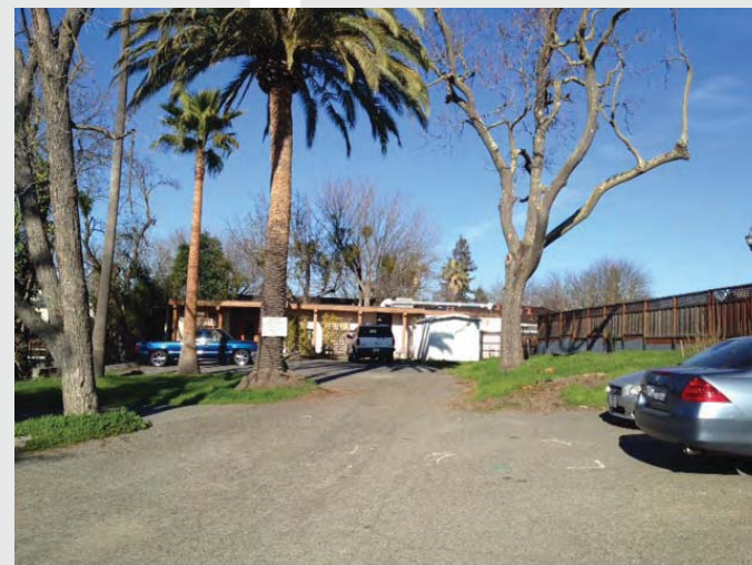
VIEW OF (E) STRUCTURE
