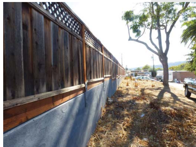
VIEW OF (E) FENCE @ EAST P.L.
