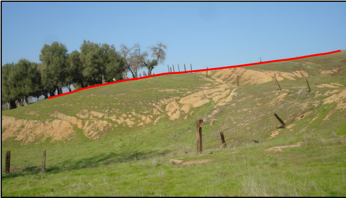
Figure 8: Existing Cut and Slope
