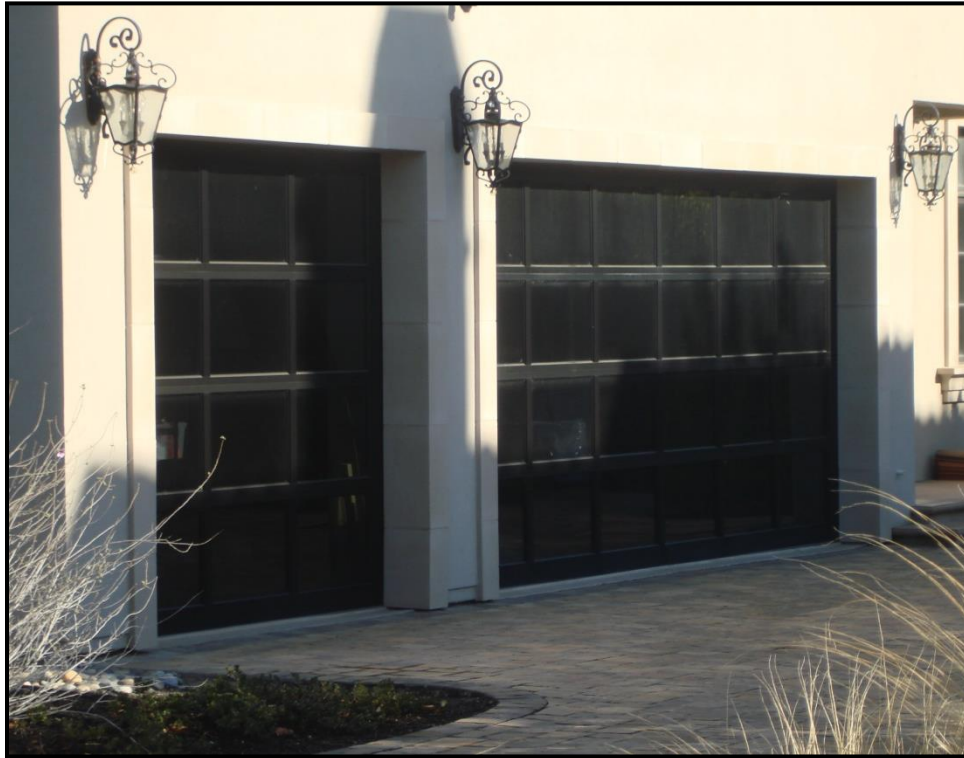
Figure 13, Glass Garage Doors on 3724 Selvante Street.
