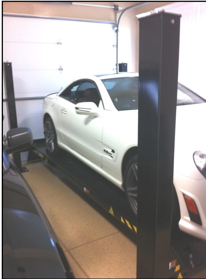
Figure 12, Car Parking Lift at 1225 Lozano Court.
