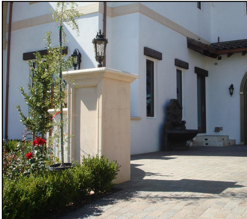
Figure 6, Column (pilaster) on South Side of Auto Court Entrance.
