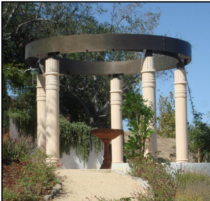
Figure 18, Partially Constructed Gazebo
