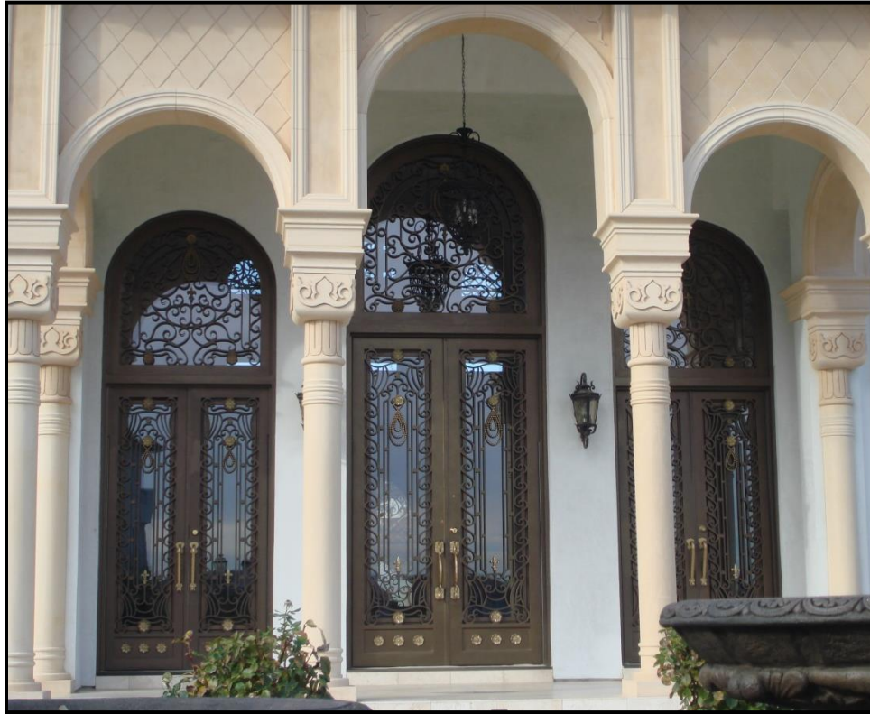
Figure 15, Front Entrance Doors and Porch Area.
