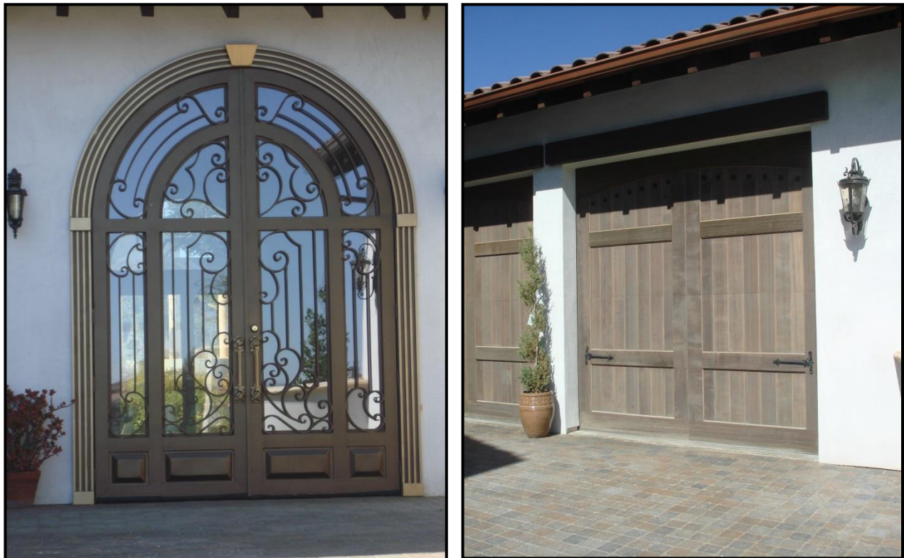
Figure 11, Glass Garage Doors on Garage 1 and Solid Garage Doors on Garage 2.
