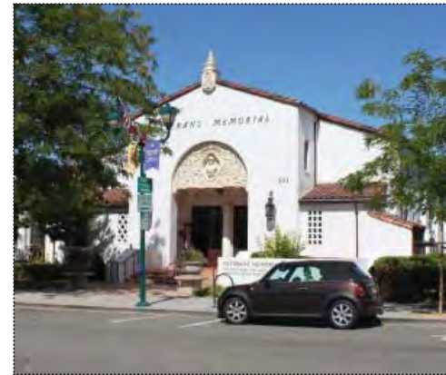
The Veteran's Memorial Building at 301 Main Street was built in 1933 (ARG, June 2012).
