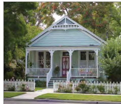
End gable residence at 4362 Second Street (ARG, June 2012).
