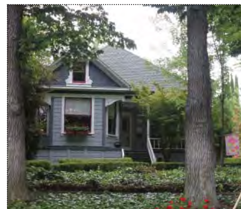
The Charles Bruce House was built at 4636 Second Street in 1894 (ARG, June 2012).
