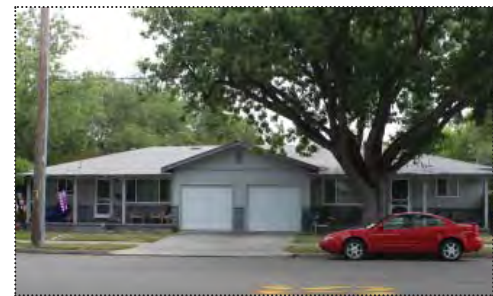
Post-war residence at 104 Abbie Street (ARG, June 2012).
