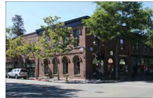
The brick building at 438 Main Street used Remillard brick (ARG, June 2012).
