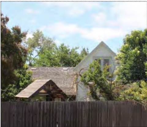
3988 First Street (ARG, June 2012).
