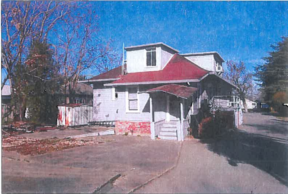
Rear (south) façade with utility room extension, porch, and dormers. View to northwest
