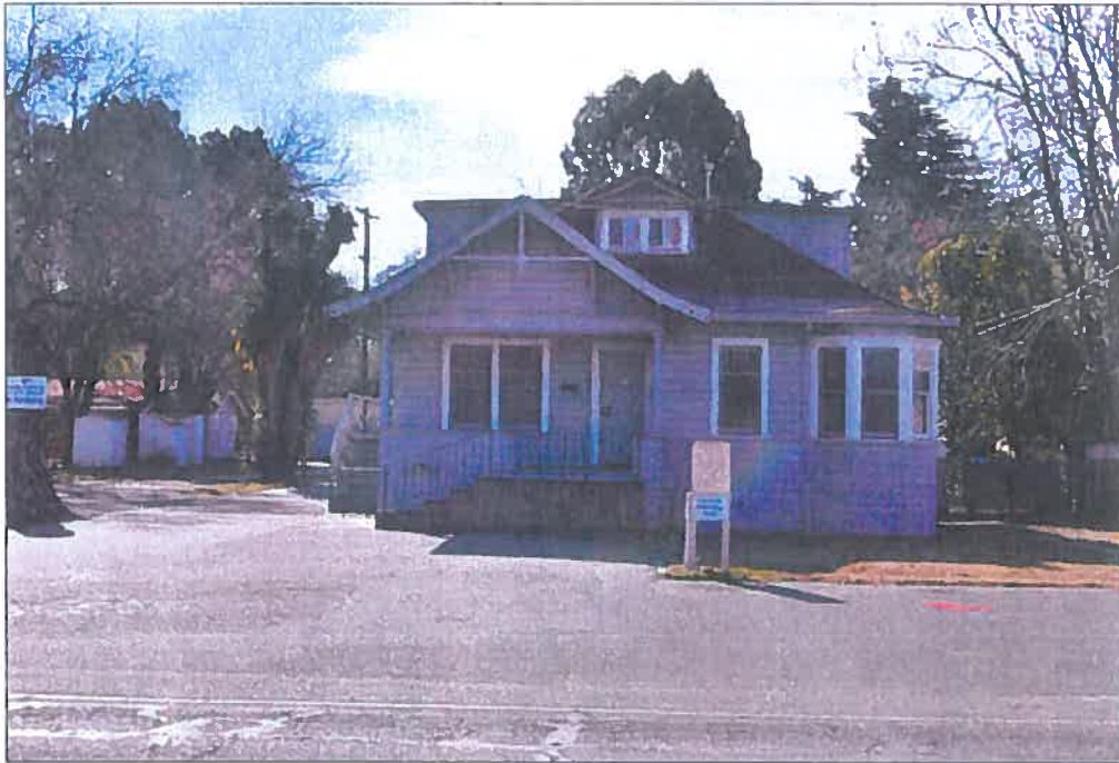
North facing front façade showing porch and asphalt covered parking area. View to south
