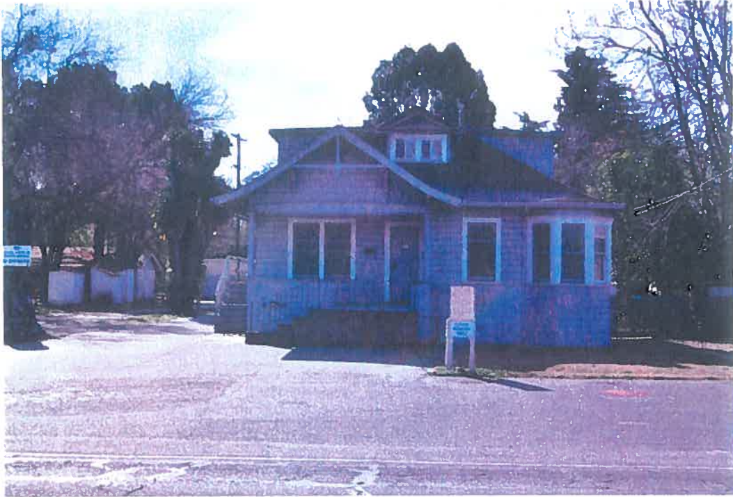
Figure 8: North facing front façade showing porch and asphalt covered parking area. View to south
