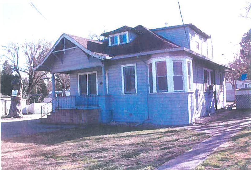
Figure 9: North facing front façade with projecting angled bay and second floor dormers. View to southeast
