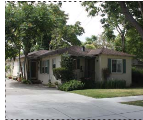
Multifamily dwelling unit at 4388 Second Street (ARG, June 2012).
