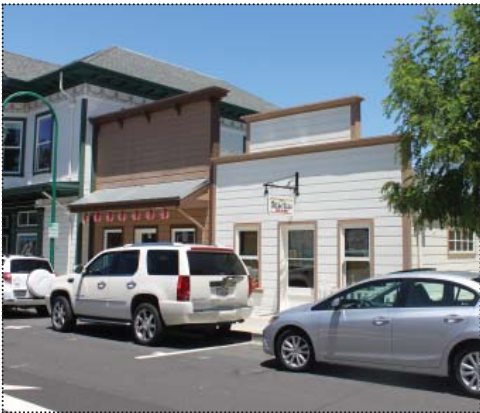
Pinkley Tin Shop was moved to the rear of 600 Main Street. The rear portion was demolished and reconstructed in 2004 (ARG, June 2012).
