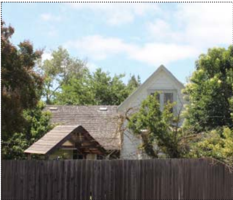
3988 First Street (ARG, June 2012).
