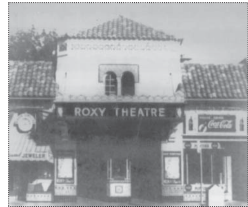
The New Lincoln/Roxy Theater was built at 641 Main Street in 1927 and converted to retail use in 1955 (from Pleasanton . Images of America, 98)
