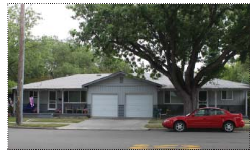
Post-war residence at 104 Abbie Street (ARG, June 2012).
