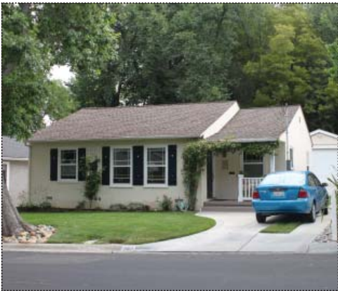
An FHA Minimum House at 360 East Angela Street (ARG, June 2012).
