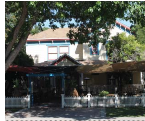
Former Jerome Arendt House at 625 Main Street (ARG, June 2012).
