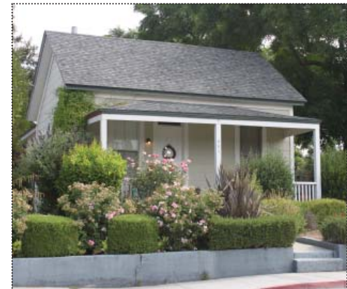
The residence at 204 Kottinger Drive is an example of a vernacular house form.
