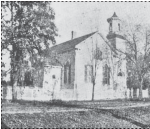
The First Presbyterian Church was built in 1876. The foundation was made of Pleasanton Company bricks (from Pleasanton . Images of America, 51).
