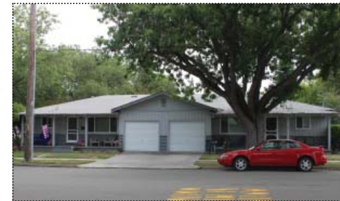
Multifamily dwelling unit at 104 Abbie Street (ARG, June 2012).
